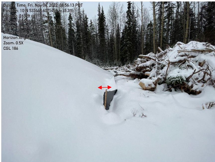
Photo 6: KP186+720 - Sediment fence installed protecting stockpile not to specification.
