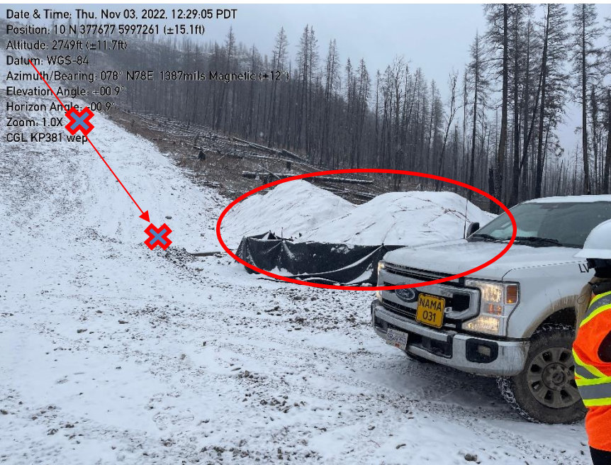
Photo 11: KP381+520 to 381+575 - Lack of rock lined feature (indicated by red arrows), straw wattles, sediment fences (indicated by red x's) and unapproved stockpiles (indicated in red circle).
