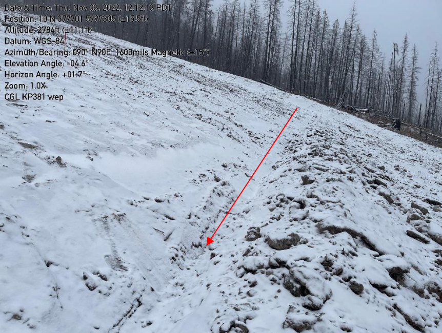
Photo 10: KP381+440 to 381+575 - Five water bars located along slope not constructed to specification.
