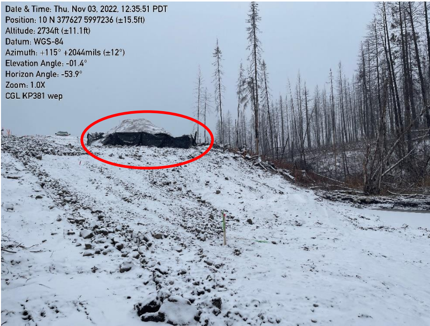
Photo 15: KP381+625 - Unapproved stockpile located on slope
