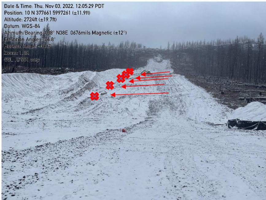
Photo 9: KP381+440 to 381+575 - Missing five correctly installed straw wattles and sediment fences.
