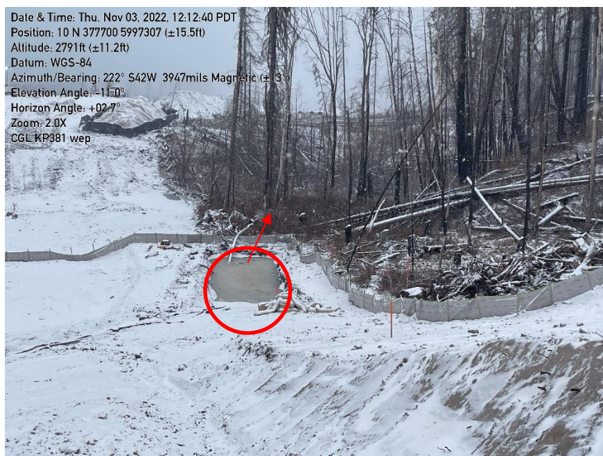
Photo 13: KP381+580 - Unapproved pumping from sump.
