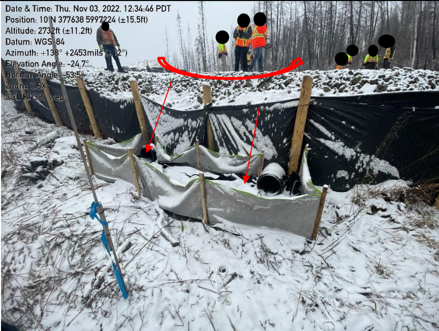
Photo 14: KP381+600 - Culvert flume outlet lacking straw wattles.
