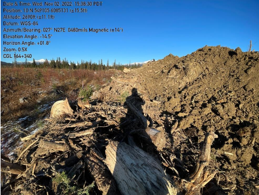
Photo 5: KP164+311 - Lack of sediment fence located behind stockpile.
