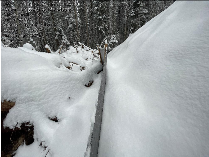
Photo 7: KP186+740 - Sediment fence installed protecting stockpile not to specification.
