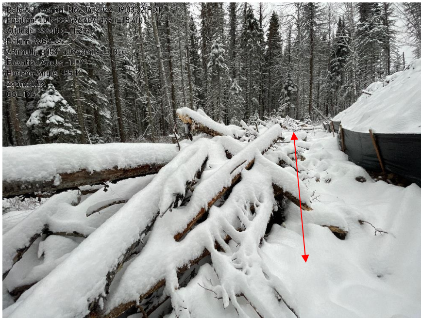
Photo 8: KP186+740 - Lack of perimeter ditch behind stockpile.
