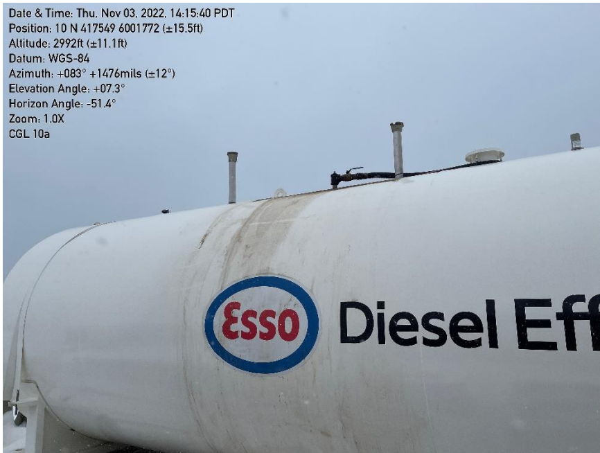
Photo 2: Spill residue on fuel tank at 10A laydown.
